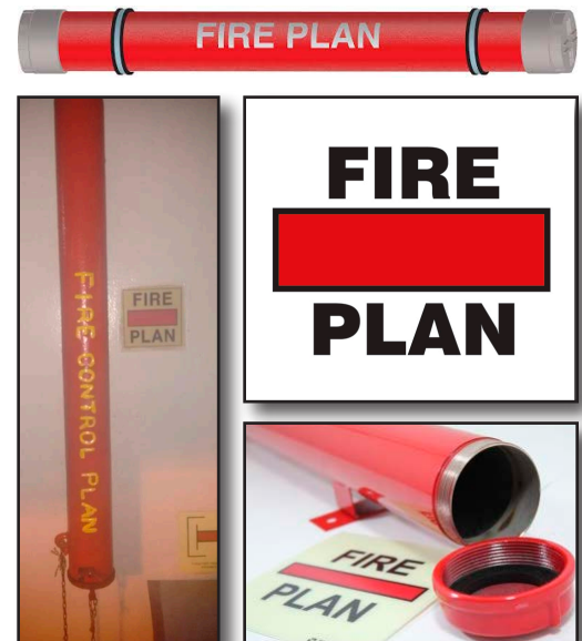
Figure 35-46 Fire Control Plans are required by U.S. Regulations as well as many other countries. Obtaining and reviewing the fire control plan must be made a priority by first arriving companies prior to initiating fire attack operations.
