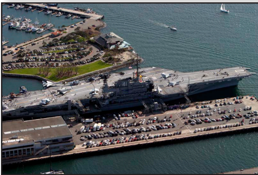
Figure 35-17 B Street Cruise Ship Terminal (top), Broadway Pier (middle), Navy Pier (bottom).
