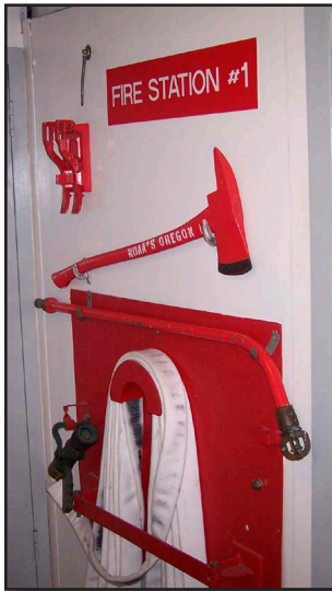
Figure 35-45 In the maritime industry, a “fire station” is merely an area staged with hose, FDC, and firefighting equipment.
