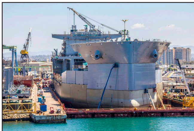
Figure 35-4 Graving Dock at NASSCO Shipyard
